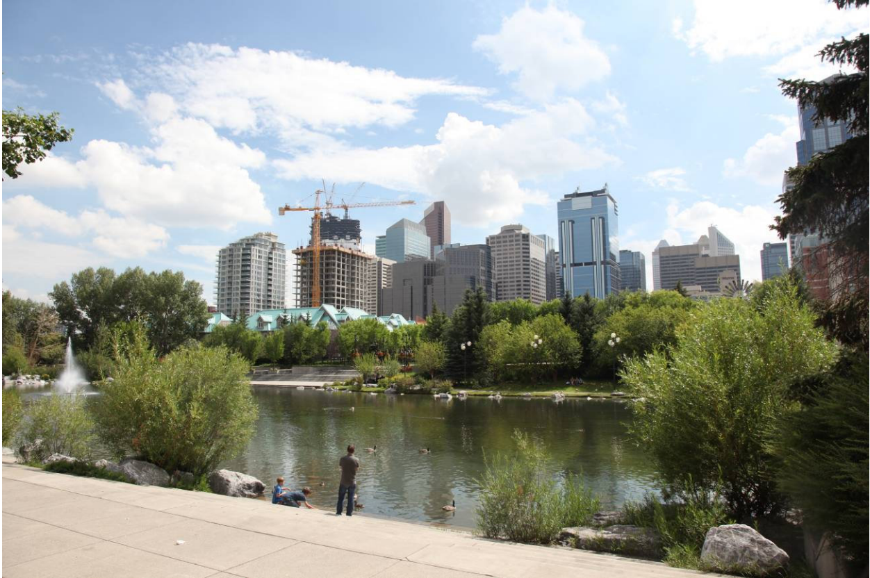
Calgary , August 2010 (Elvin Wyly). The tower under construction in the distance at left is the 58-story Bow, future corporate headquarters for the giant energy firm Encana Corporation. The Calgary urban region grew by 109 thousand people between 2001 and 2006 -- a growth rate more than twice the expected proportional rate. Calgary benefitted from “the rise in demand and prices for most commodities” that helped most of Alberta as well as Newfoundland, and it also benefitted from the expansion of the financial services sector in large centers in Western Canada. Richard Shearmur (2009). Growth in the Canadian Urban System, 2001-2006 . Montreal: INRS, p. 2.
