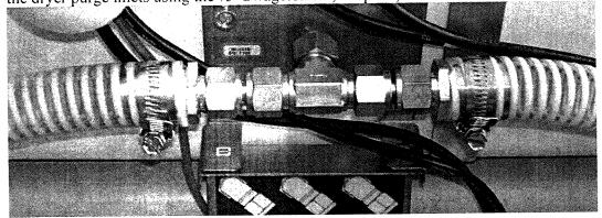
Connect the other end of these 1" hoses to the dryer purge inlets as shown below.
